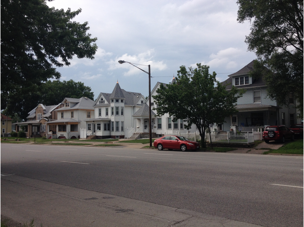
Figure 1. A row of houses line 7th Avenue, one of the busiest streets that runs through the KeyStone neighborhood in Rock Island. Historic houses showing deterioration like several of these is typical of Rock Island.
