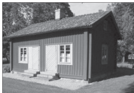
A typical old house in Fellingsbro.
