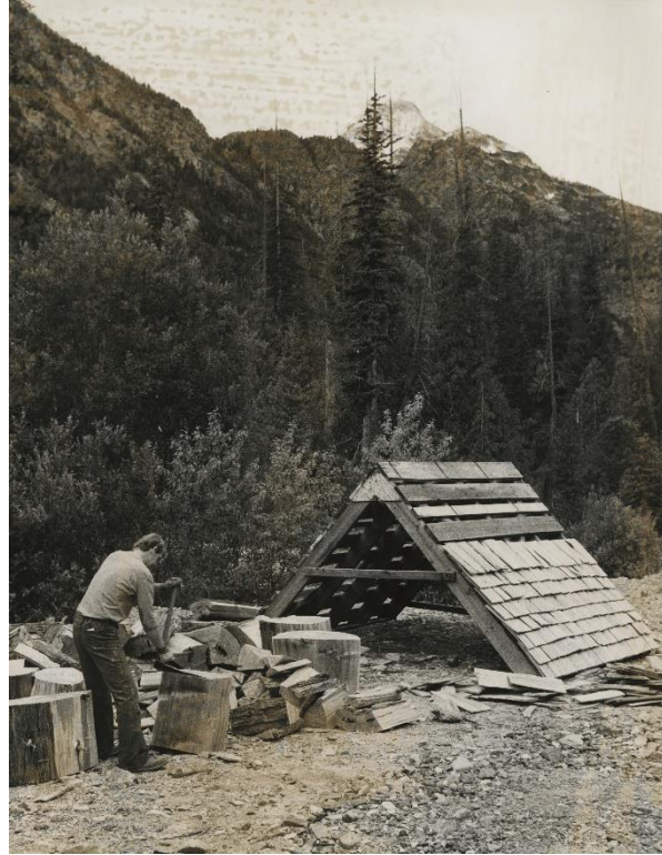
Figure 4. Villager of Holden Village cutting wood shakes for a roof. Erwin Weber. Holden I Copy, No. 4, in MS 112 Weber (Erwin) Papers circa 1930s-2000s, Special Collections, Augustana College, Rock Island, Illinois: 91.
