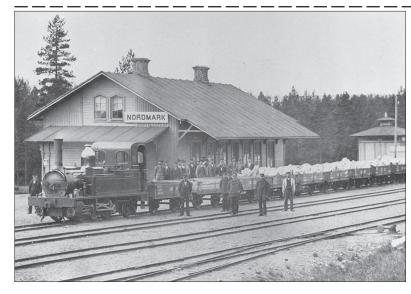
This train is seen by the Nordmark railway station in Värmland around 1900. The train is transporting limestone from the limestone mine to one of the local blast furnaces (masugn), where it was used in the process of ironmaking.
