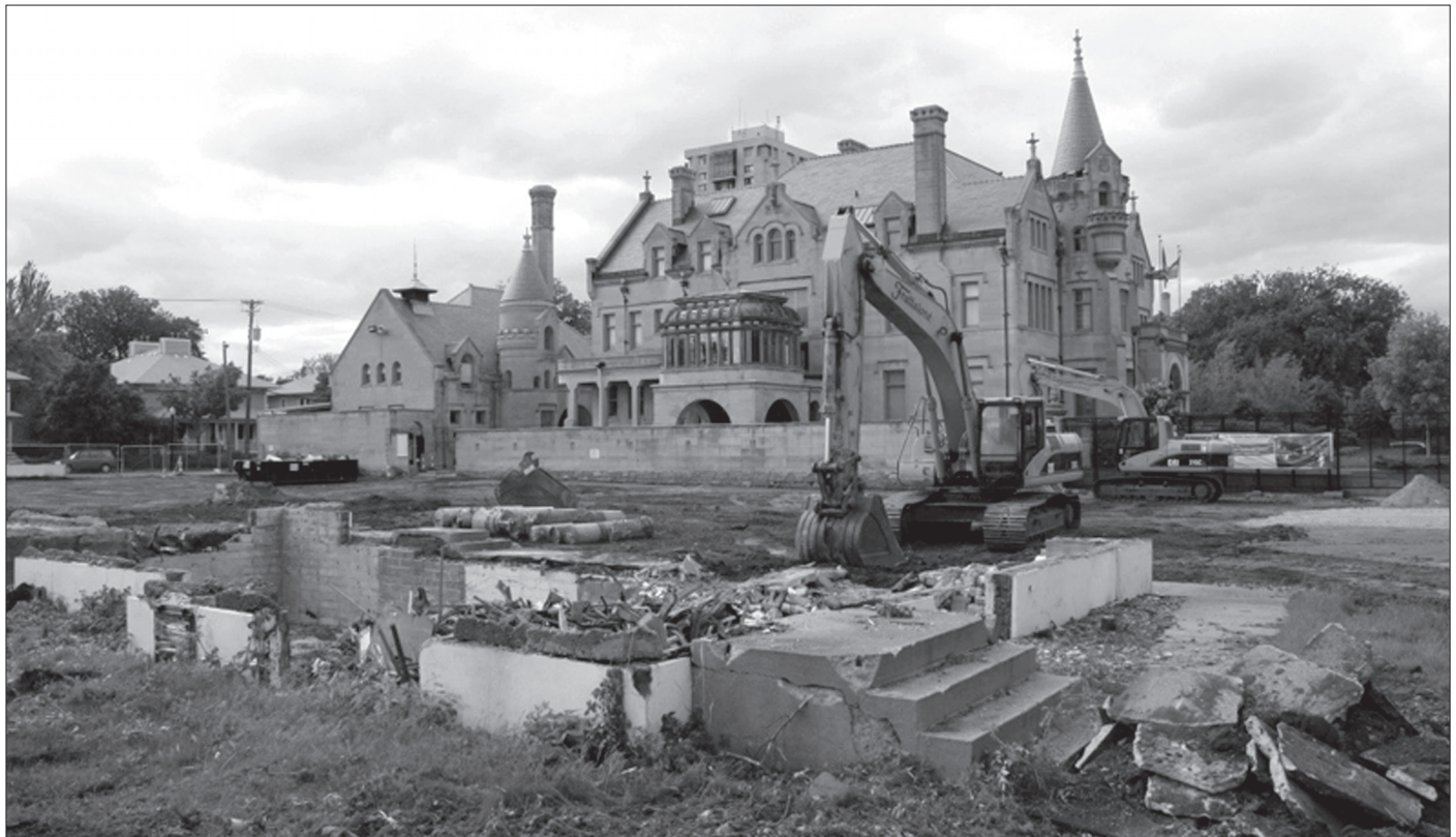
Picture from < http://www.americanswedishinst.org/ASI/Home.html > showing the state of construction on May 30, 2011.
