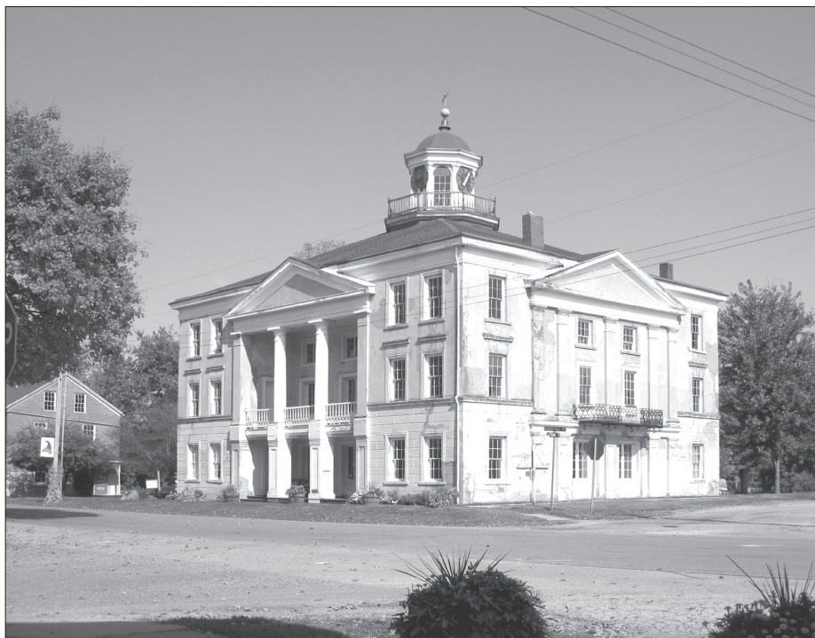
The Steeple Building, (Tornbyggningen), site of Bishop Hill Heritage Association archives. Photo: E.Thorsell 2010.
