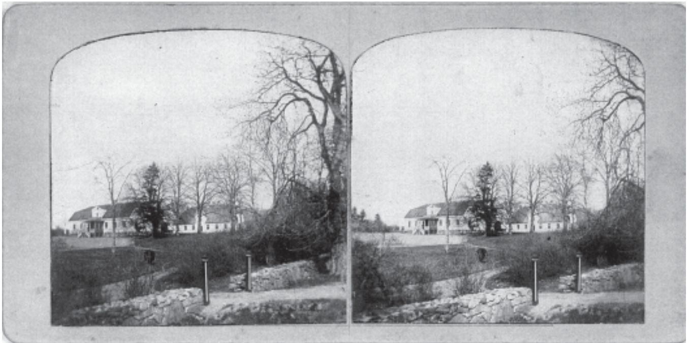
Stjärnarp – manor house and stable block, Eldsberga parish in Halland, ca. 1870–1890.
