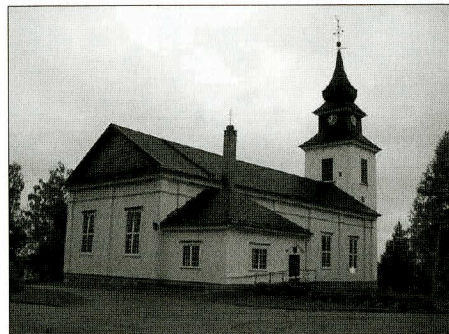
Wilhelmina church in Västerbotten, Sweden.
