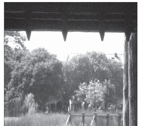
Entrance with portcullis.
